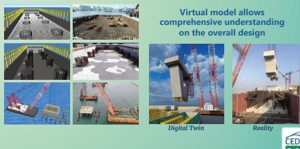
Digital twin for the design of precast V-piers
